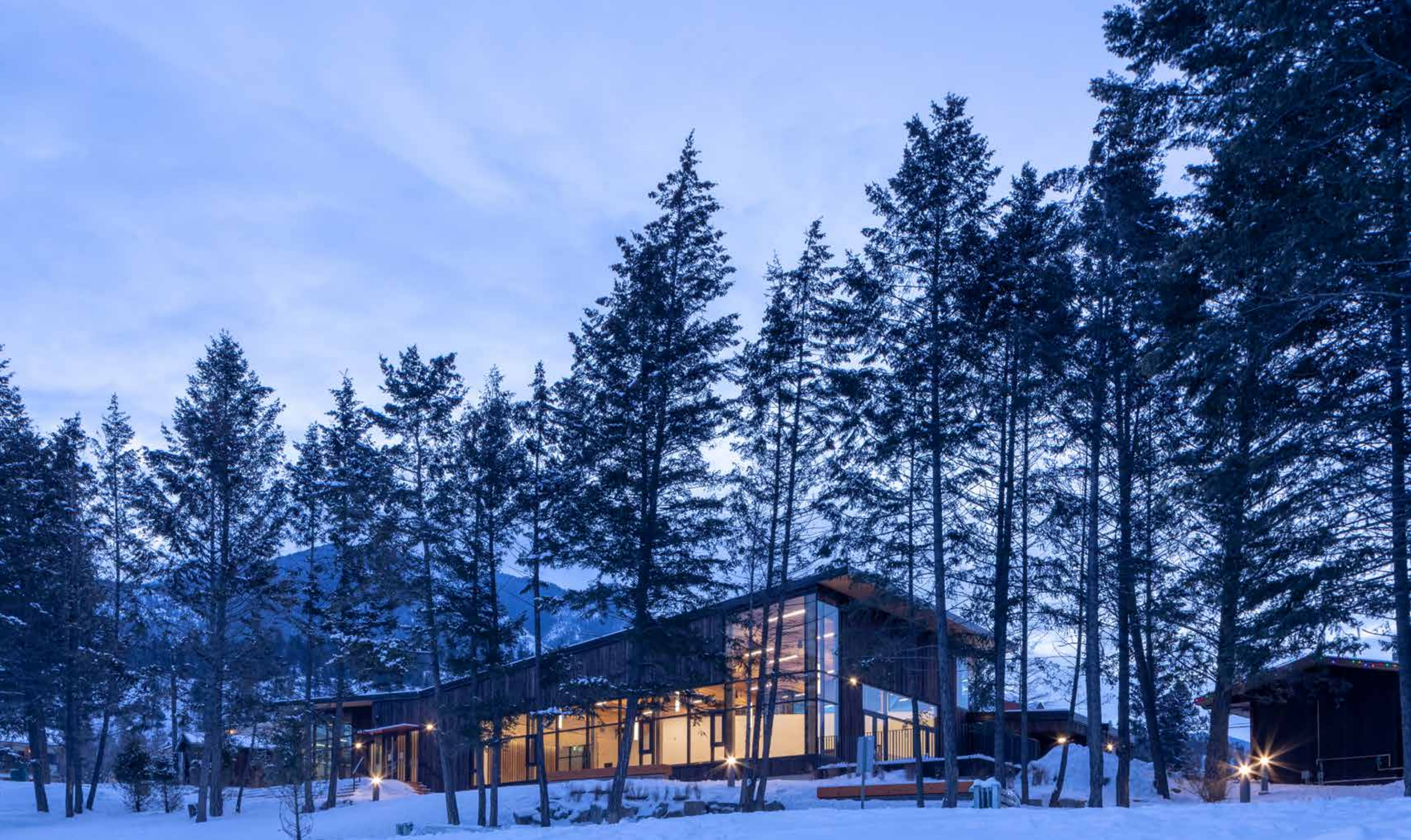
Radium Hot Springs Community Hall + Library
